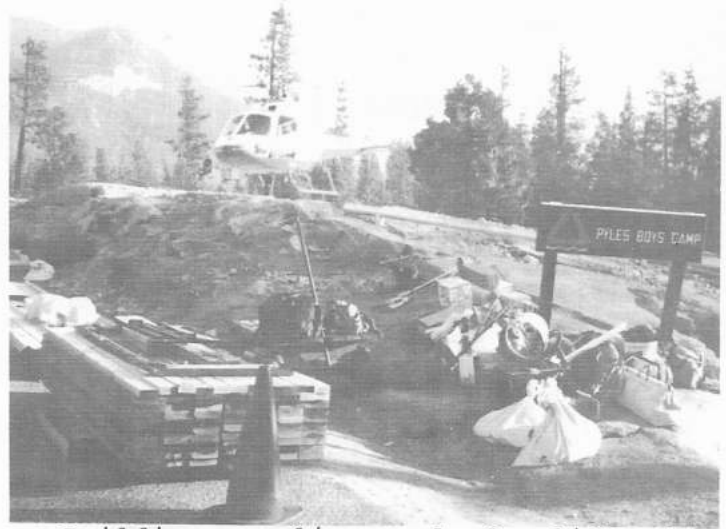
Building supplies ready for lift off
