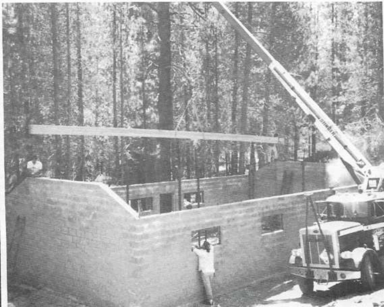
50 ft. long beams are lowered to Kybo
