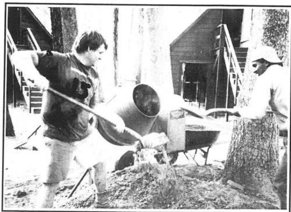
Spuds and Dolphin had mix concrete for the sidewalk construction
